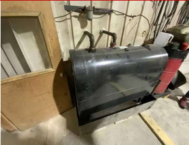
13 - OIL STORAGE TANK
