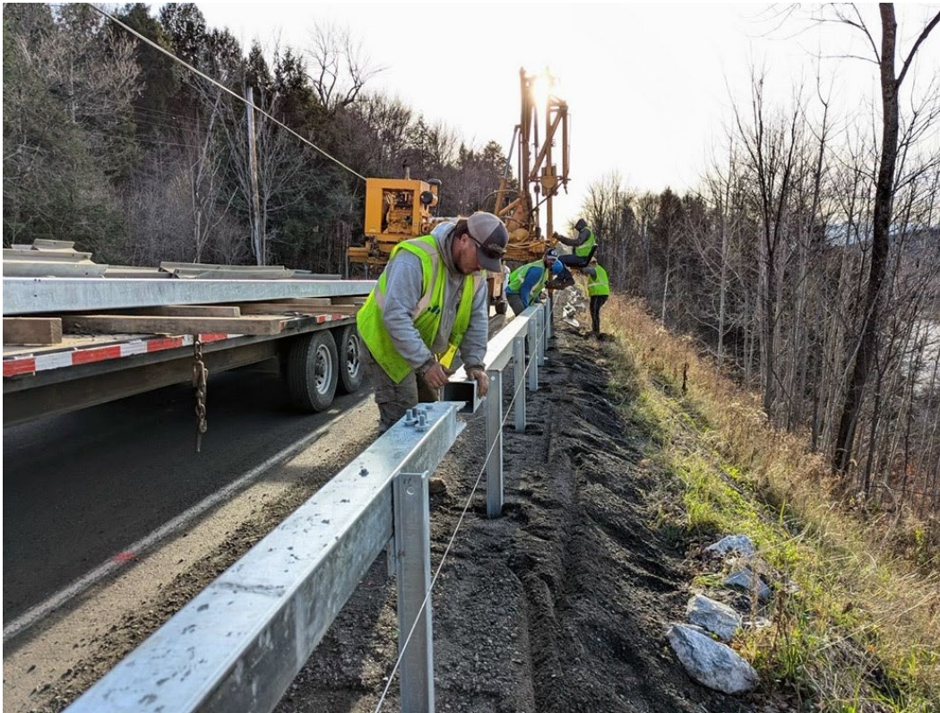
Crews install guardrail on VT 15.
