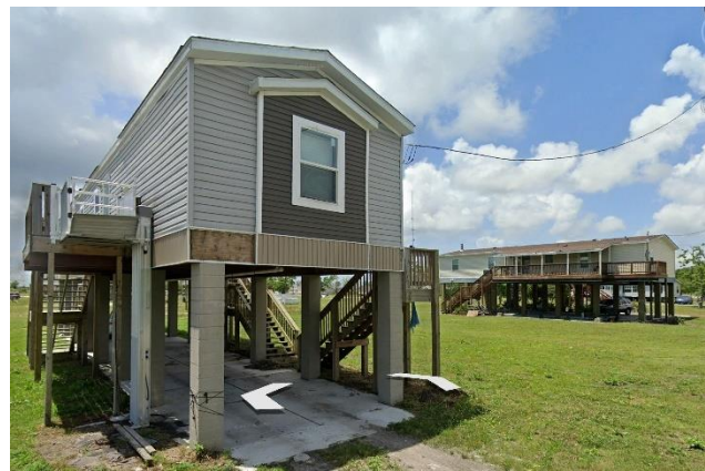
Views of Ironton, summer of 2022. The only remaining houses are the few that were elevated on piers in the years following Katrina, and a handful of temporary trailers. The gaps between houses mark the locations of the houses that were destroyed by Hurricane Ida. Source: Google Earth.
