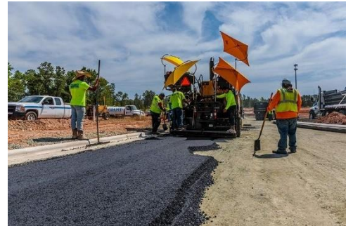
Street paving in progress. Source: https://giantdevelopmentinc.com/services/subdivision-paving
