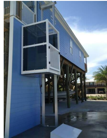
An example of an elevated house with a covered lift.
