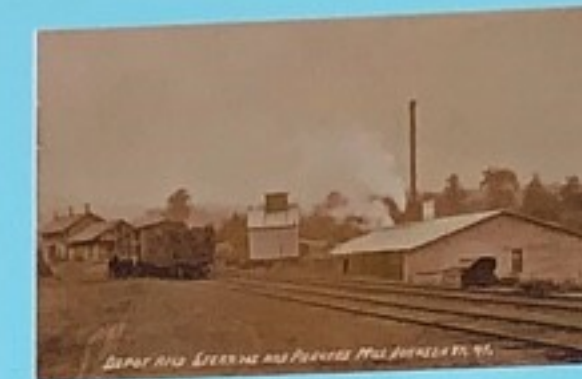
Train station and rail yard with siding servicing Parker & Stearns hard wood flooring mill.
