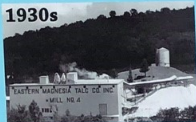
Site visible from Rail Trail. The water silo on the hill served as a reservoir for sprinkler systems. Waste pile would be later reprocessed by flotation process.
