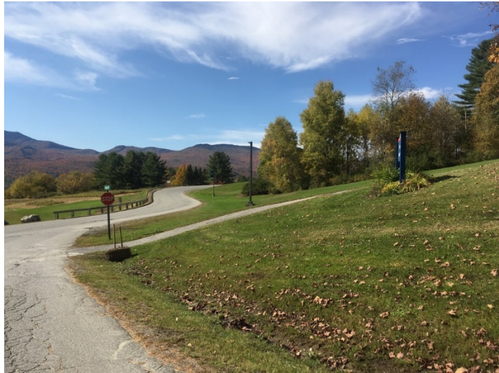
Figure 8. A grass swale transports stormwater to the intersection with College Hill, where an infiltration trench is proposed.
